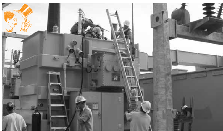
Substation crew replacing transformer bushing.
